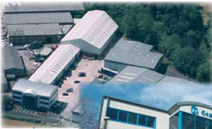
Cembre Ltd. factory in Curdworth (Birmingham)
